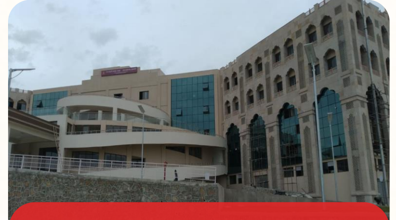
Hospital Project In Udaipur Rajasthan
